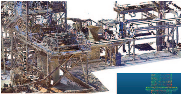
EXISTING PIPING INSTALLED ONSITE WITH A 3D MODEL OVERLAY OF THE REPLACEMENT SPOOLS
